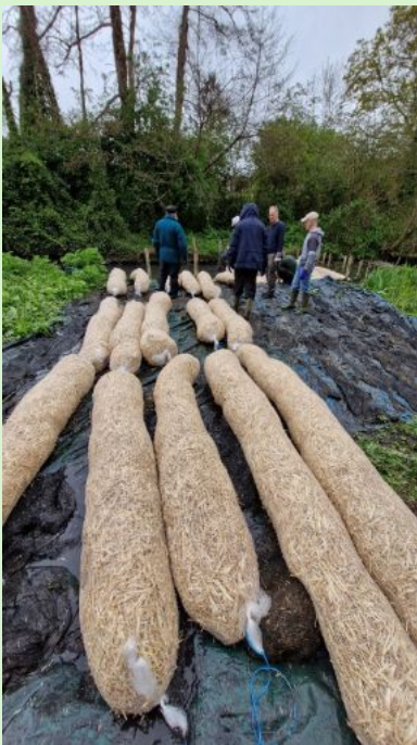
The New Barley Straw Bales installed at the lake Inlet.
