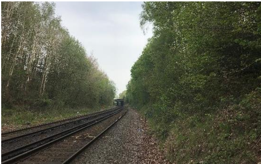
Image 2. View north from Wokingham Station to Reading road bridge.
